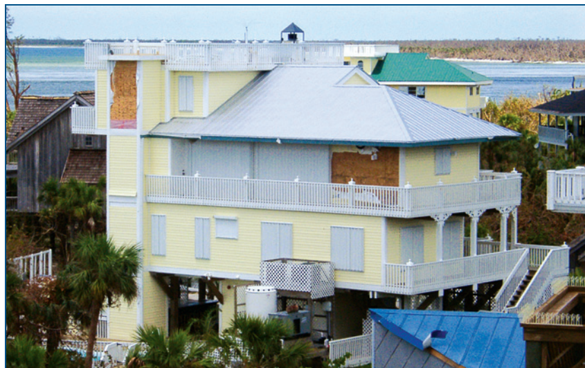
FIGURE 2-3: Building built to the 2001 Florida Building Code (FBC) standards with no structural damage after Hurricane Charley (North Captiva Island, 2004) (SOURCE: FEMA 488)
